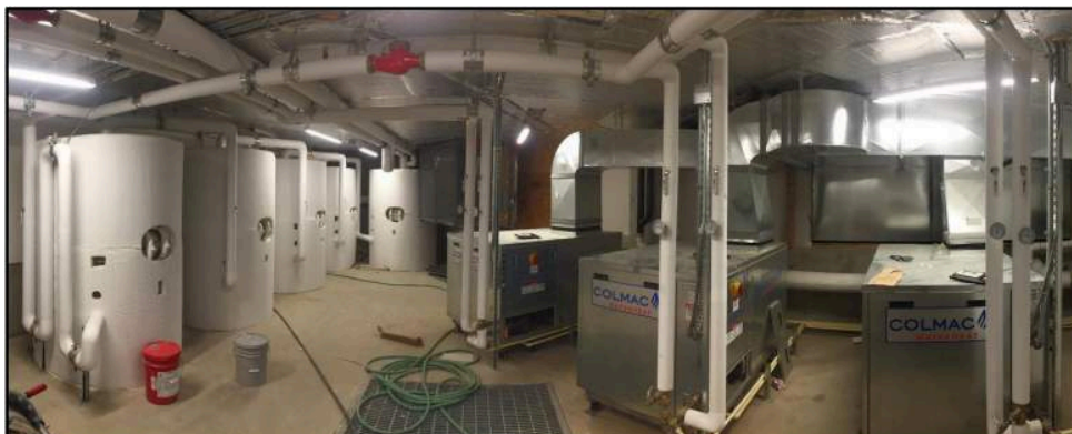
Figure 14: Ecotope Case Study "RCC" system for 194 unit Multifamily building, using best practices in central heat pumps for domestic hot water, from ACEEE presentation by Shawn Oram.
